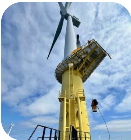
As a Red Seal Electrician Etienne de Kock exchanged his proudly Africa Skills PPE for protective and safety gear as a high-voltage electrician in the Netherlands. Photo: Supplied
