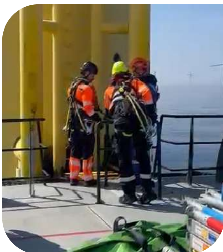
25-year-old Africa Skills Red Seal Electrician Alumni Etienne de Kock on duty as a high-voltage electrician installing and maintaining Offshore Wind Power on the ocean at the Netherlands. Photo: Supplied
