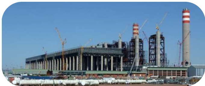
Medupi Power Station, Ellisras, Limpopo in South Africa. Photo: Wikipedia
