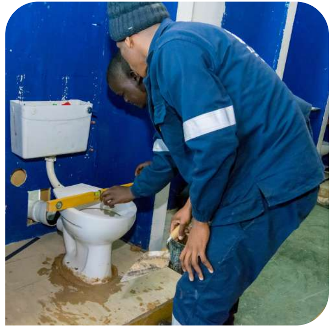
Precision bathroom installations form a key foundation in mastering essential plumbing skills. Photo: UXi AD Media
